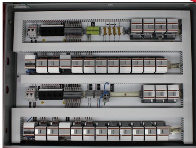
Figure 3. Distributed I/O can share signals between other peer distributed I/O systems from the same vendor or alternative vendors using industry open or standardized protocols.
