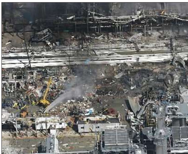
Figure 2. Aftermath of the 2005 explosion at the BP refinery in Texas City, Texas. Courtesy: U.S. Chemical and Hazard Safety Investigation Board
