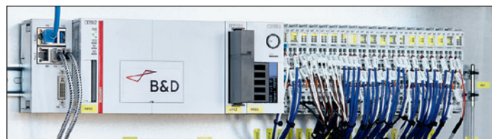
Figure 4. The CX2062 Embedded PC with the attached EtherCAT Terminals forms a powerful and compact control solution for the measurement and analysis system. Courtesy: Beckhoff
