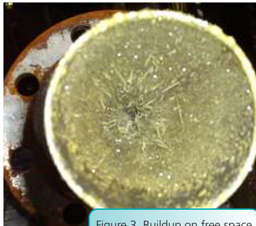
Figure 3. Buildup on free space radar antenna, which does influence the safety function.
