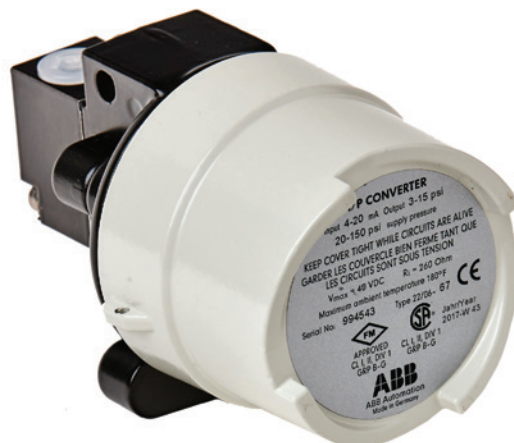
Typical I/P used in a remote mount application.
